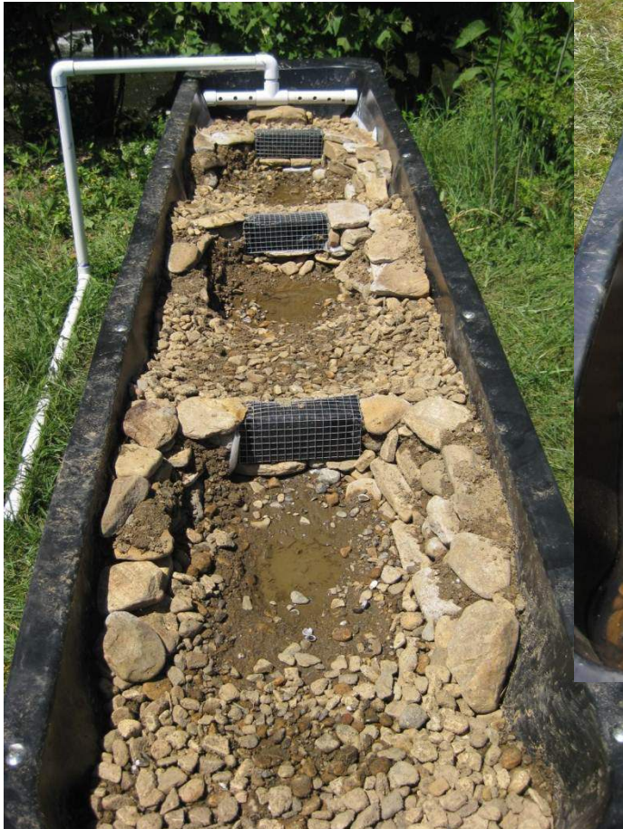
ROCK DROP STRUCTURE
