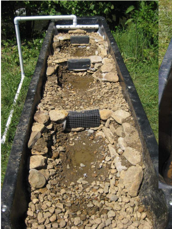
ROCK DROP STRUCTURE
