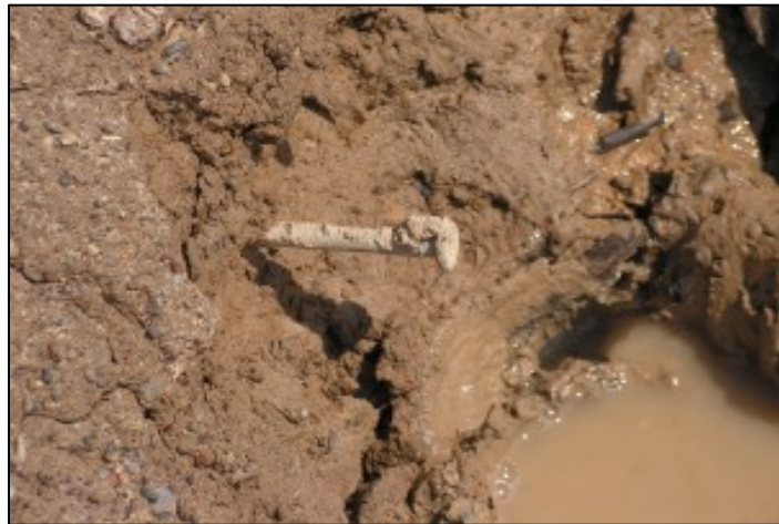
An erosion pin like the one shown in this photograph is a common way to measure active soil loss on a river bank. The metal rod is set into the bank with a portion sticking up above the surface. The length of the pin above the surface is measured and monitored over time.
