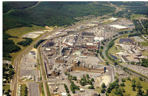
An aerial photo shows the former DuPont plant. The South River is on the right side of the photo.
