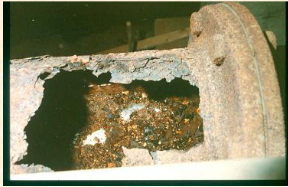
Metallic mercury in gravel-filled pipe
