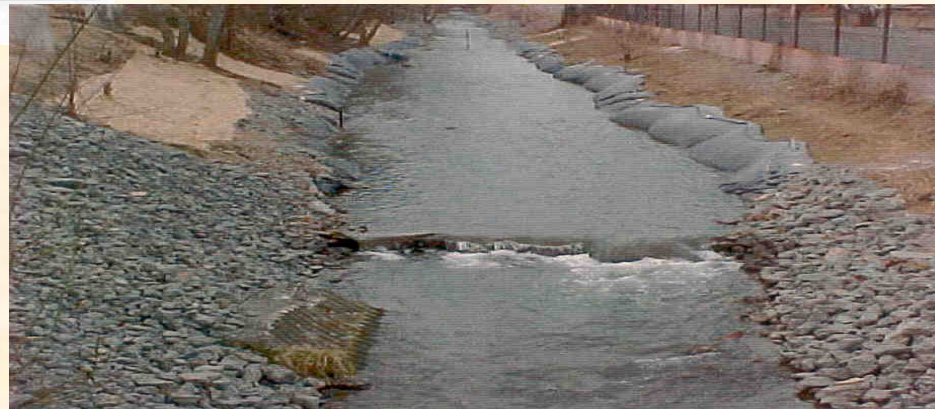
Fig. A.6. UEFPC Bank Stabilization final site with riprap and geotextile tubes filled with sand.
