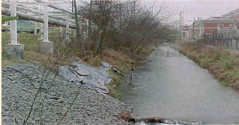
Fig. A.1. UEFPC Bank Stabilization site before construction.
