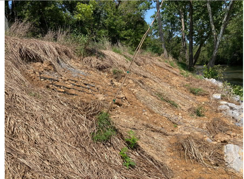
Photo 2 - Bank Erosion at Top of Bank
