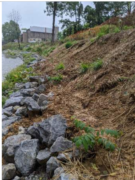
Photo 3 - Sloughed Material on Stone Toe
