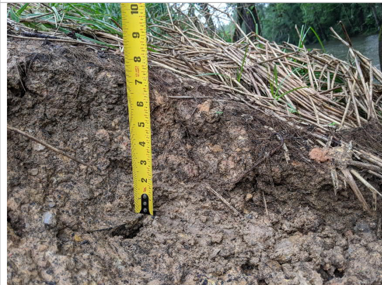
Photo 4 - Material above Geocell
