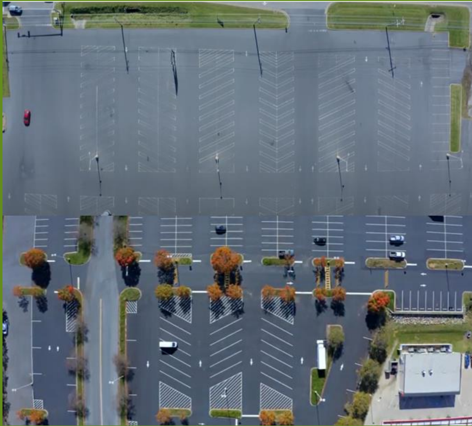
Parking lots before and after city ordinances required interior landscaped islands for parking lots. Newer lots are designed with trees to enhance the look of a property, provide shade protection, and reduce impervious surfaces.
