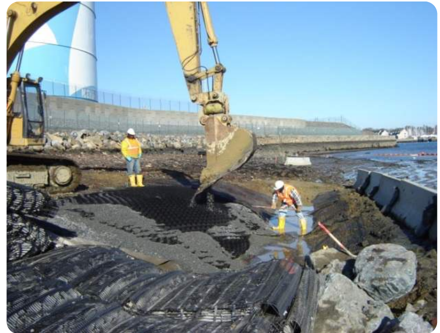
Backfilling with Blended Cover
