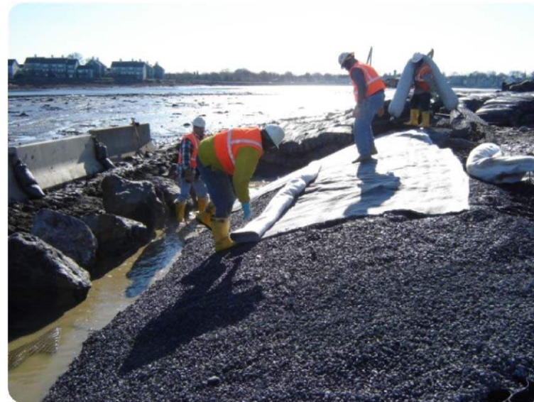
Placing Reactive Core Mat
