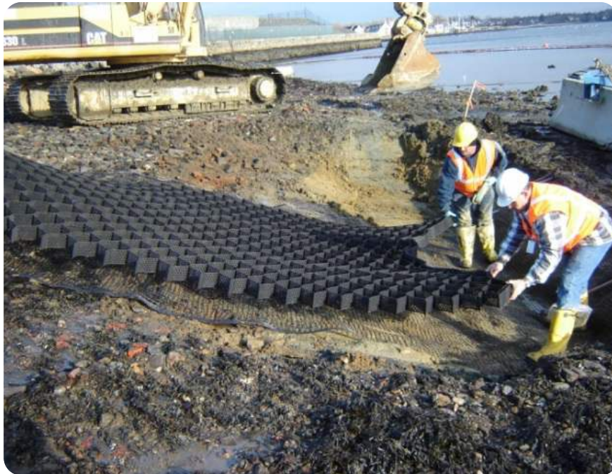
Placing Geoweb®
