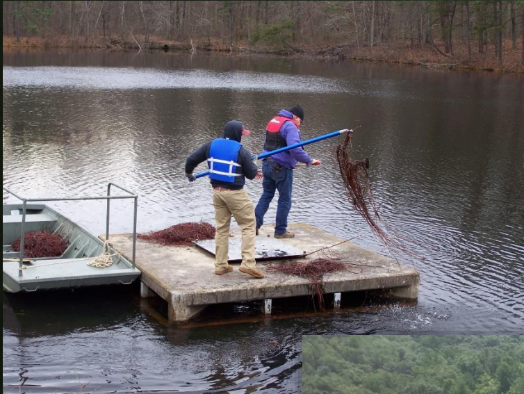
Clearing a Riser Blockage
