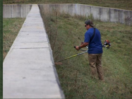
Clearing woody vegetation
