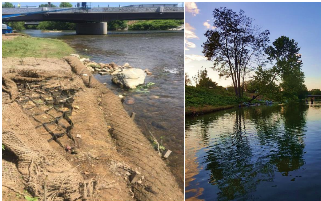
Figure 46 Implemented stabilization efforts: close up of reactive cap layer (left, AECOM & Collins, 2017) and overall implemented efforts 6 months later (right)
