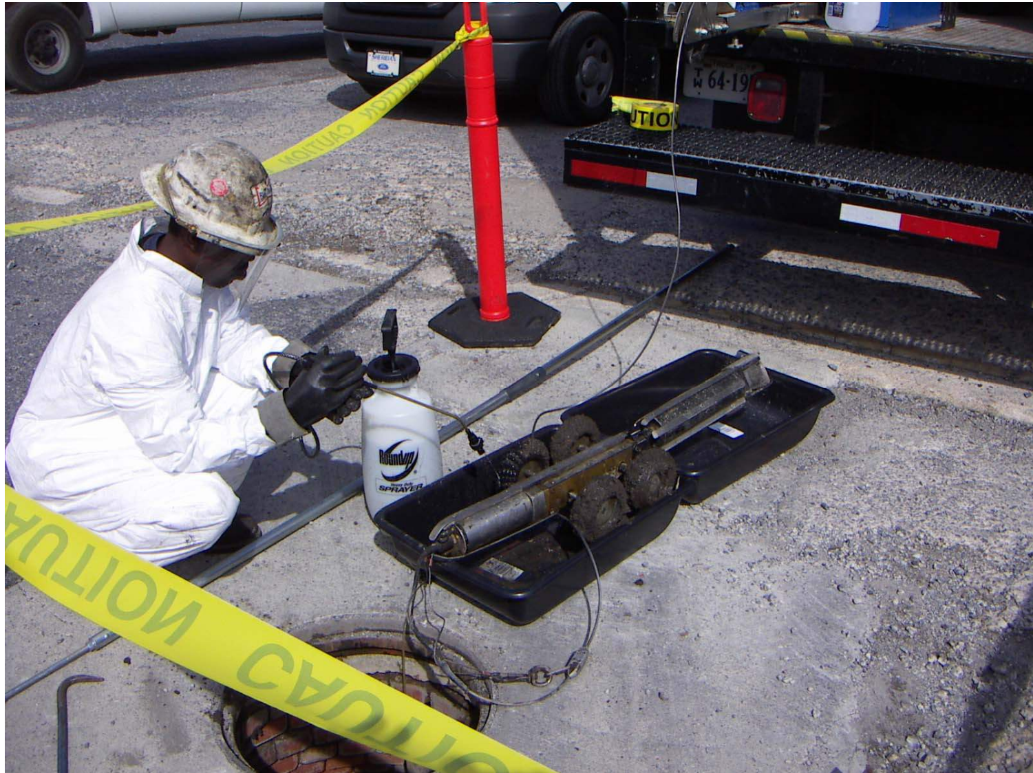
The camera was cleaned after each pipe run.
