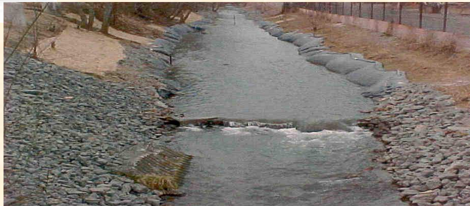
Fig. A.6. UEFPC Bank Stabilization final site with riprap and geotextile tubes filled with sand.
